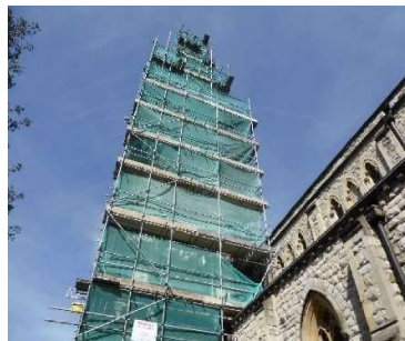
Tower fully wrapped May 2016
