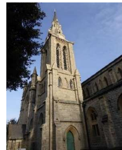
Work complete and scaffolding down, December 2016
