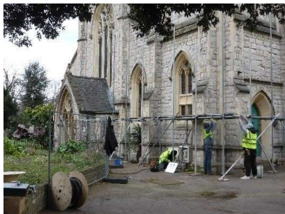
Scaffolding arrives Feb 2016
